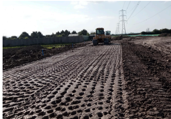
Trial embankment construction
