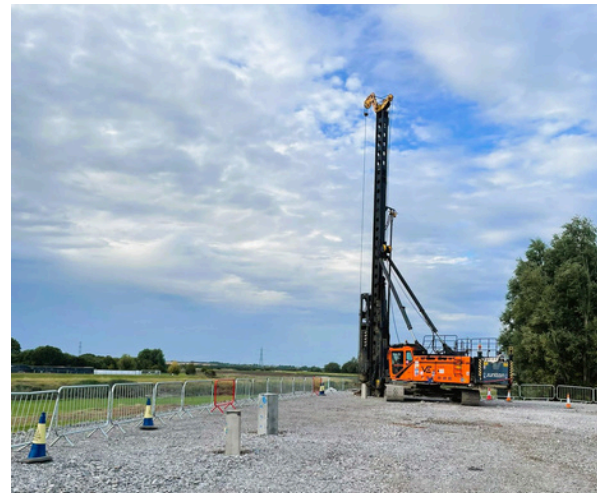
Pre-cast concrete test pile installation at Express Park (right bank)
